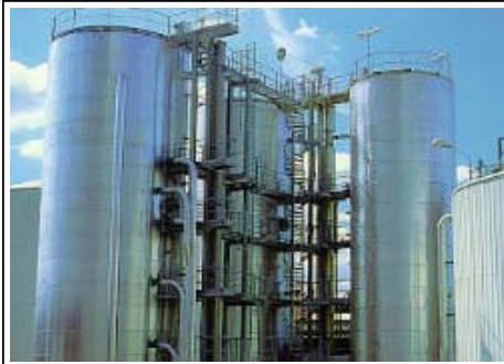
Anaerobic Reactors
