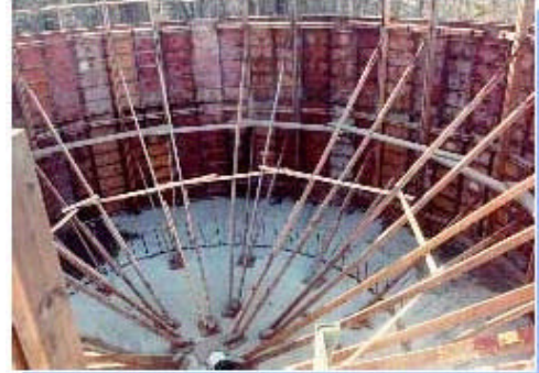
Concrete Shell Forms
