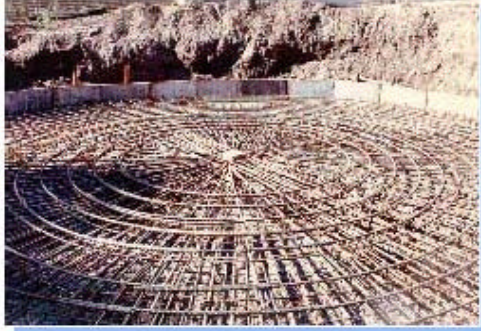
Reactor Clarifier Foundation
