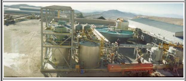
Operation since 1995, High Purity Water for Electrowinning Reactor Precipitation, Filtration, Dual Stage Reverse Osmosis
